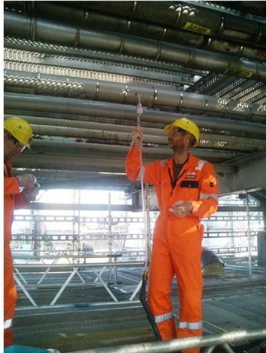
**Figure A3-10 Gas sampling during phase 2 on an operating plant.**
