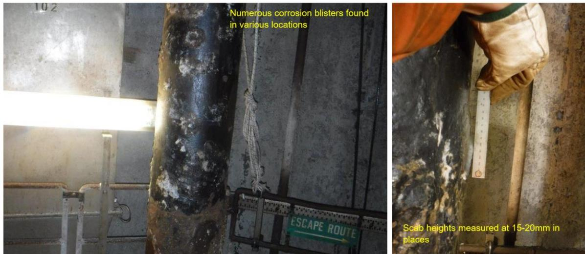
**Figure 8-13: Riser after insulation and passive fire protection removal. Numerous corrosion blisters (scabs) were found (left) with scab heights measured up to ~ 15-20mm in places.**
