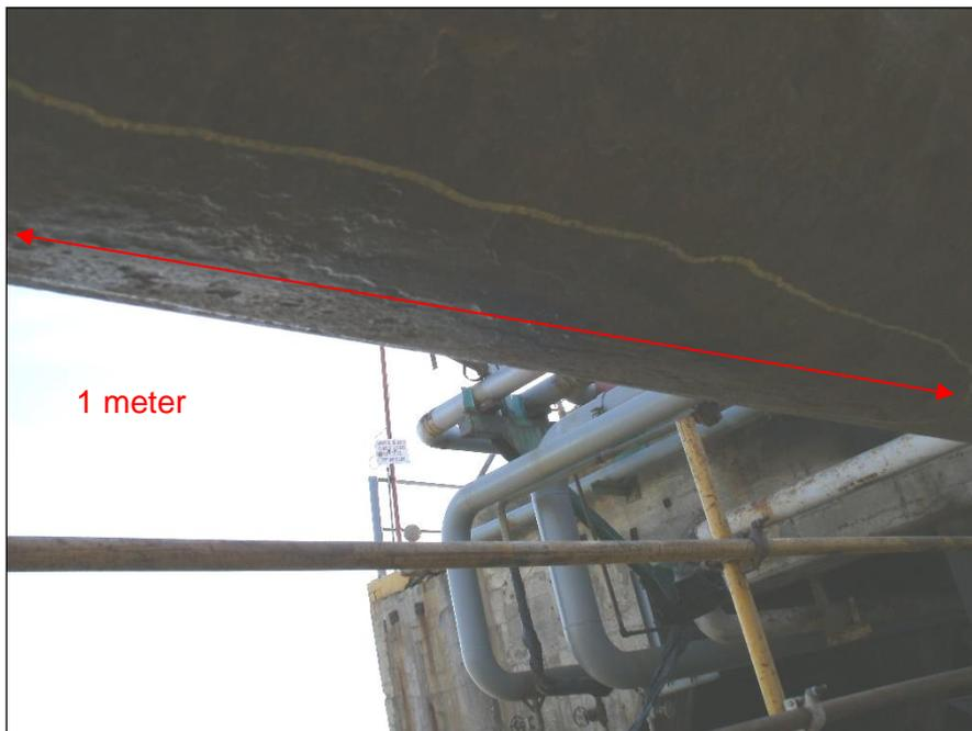
**Figure 8-10:** Corrosion detected at 6 o'clock (180°).
