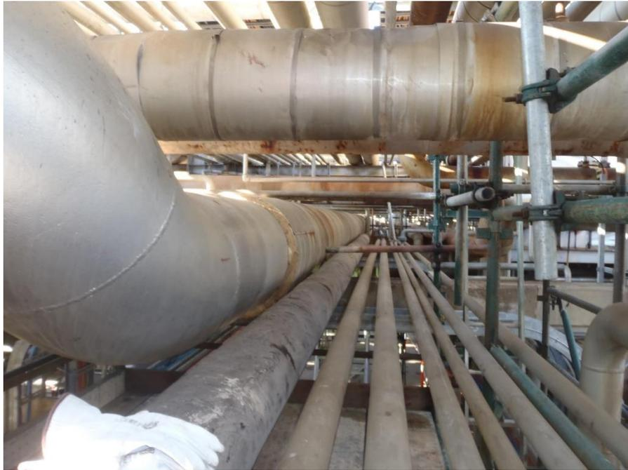
**Figure 8-6: Test location for inspection of 24" high pressure gas line.**
