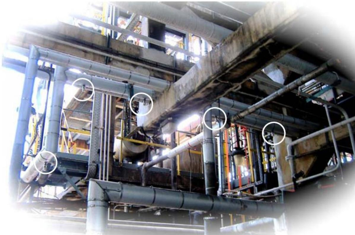
Figure A2-2: H2Obvious devices installed on a UK refinery
