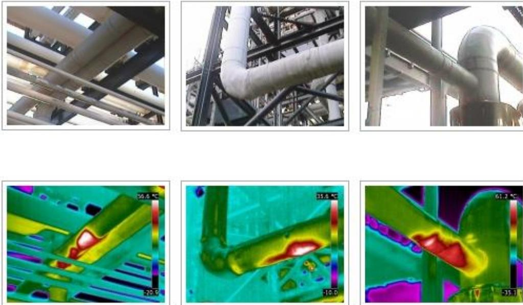
**Figure A2-6: Hot spots on areas of process pipework showing increased thermal conductivity due to moist insulation (courtesy Infrared Vision).**
