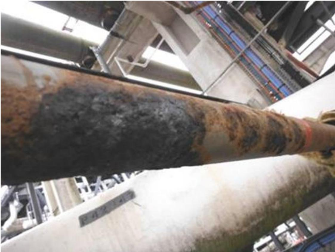
**Figure A1-4: A further example of CUI, following insulation removal (courtesy Total)**
