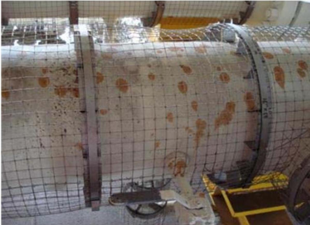
**Figure A1-1: An example of a personnel protection cage (courtesy Total).**
