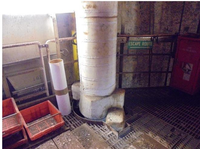
**Figure 8-11: Live gas export riser in an offshore location.**
