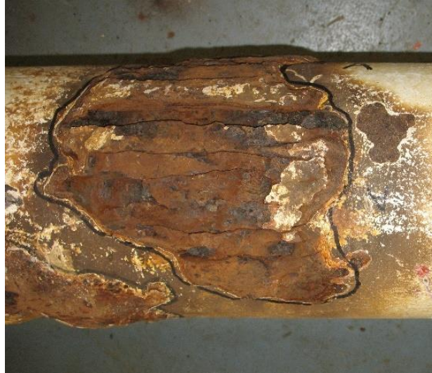
Figure A1-2: Example showing more extensive cracks in the coating and partial loss of the coating
