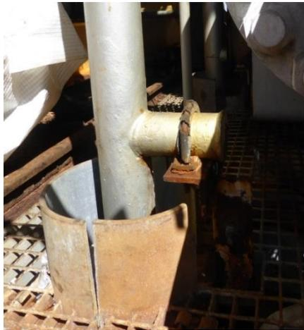
**Figure 4-1: Horizontal trunnion support on vertical pipework**
