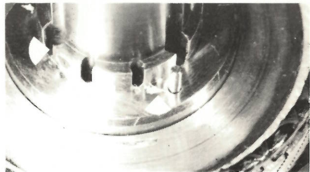
Figure 18. Sharp edges and insulation debris
